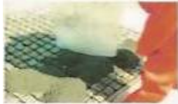
Spread material on the surface
