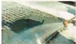
Increase density and prolong curing process by rinsing with soft jet of water
