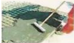
Sweep into the joints diagonally
