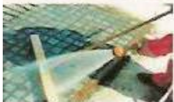
Clean the surface with soft jet of water
